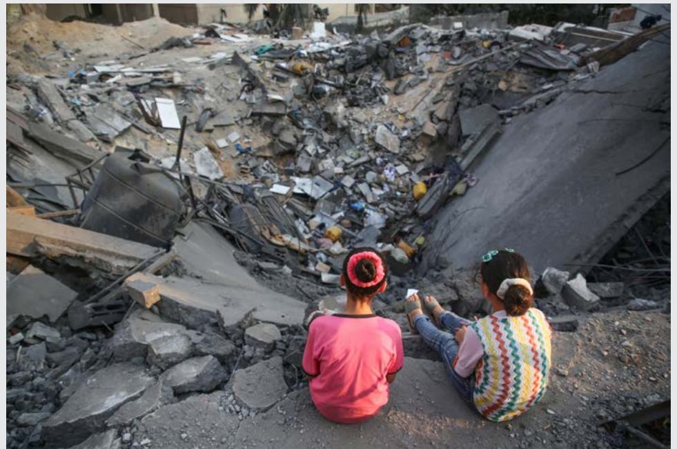
Palestinian children inspect their damaged building in Gaza city. The shattered building was once home to 17 people, including children. (Majdi Fathi/NurPhoto via Getty Images)
